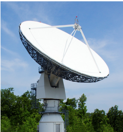
Fig. 3 The Morehead State University 21-m ground station has been upgraded with support from NASA’s Advanced Exploration Systems to become the first non-NASA Affiliated node on the DSN. Referred to as DSS-17, the station will support NASA interplanetary CubeSat missions.
