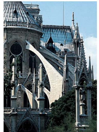
FIGURE 9–30 Flying buttresses (on the cathedral of Notre Dame, in Paris).
