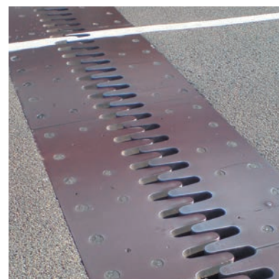
FIGURE 13–3 Expansion joint on a bridge. Note center white line of highway.
