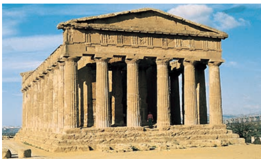
FIGURE 9–21 This Greek temple, in Agrigento, Sicily, built 2500 years ago, shows the post-and-beam construction. The columns are under compression.
