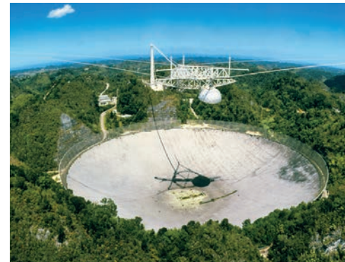
FIGURE 25–33 The 300-meter radiotelescope in Arecibo, Puerto Rico, uses radio waves (Fig. 22–8) instead of visible light.
