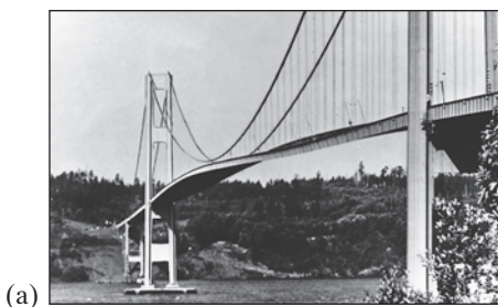
FIGURE 11–20 (a) Large-amplitude oscillations of the Tacoma Narrows Bridge, due to gusty winds, led to its collapse (November 7, 1940). (b) Collapse of a freeway in California, due to the 1989 earthquake.
