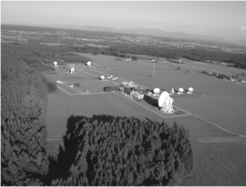
Figure 14.3 The Weilheim ground station is located on a plain, and is surrounded with forest, with the Bavarian Alps in distance. Tracking down to three degrees elevation is possible (Credit: DLR)
