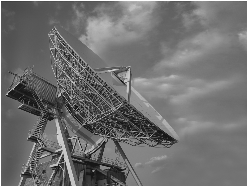
Figure 14.1 Weilheim 30 meters antenna (Credit: DLR)
